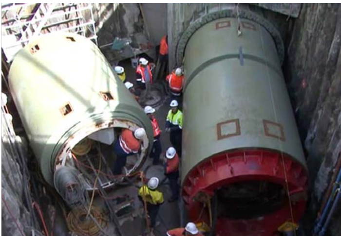
Setting up the TBM at Burrows Road
